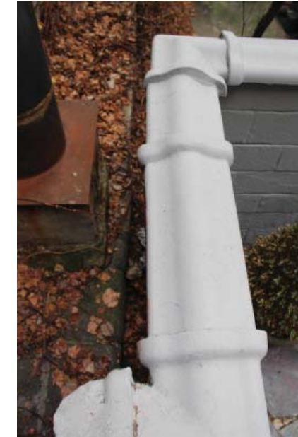
Rear yard wall at southwest
