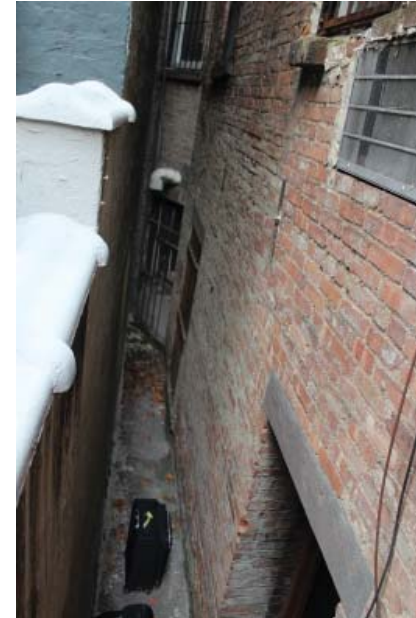
Light well to south
